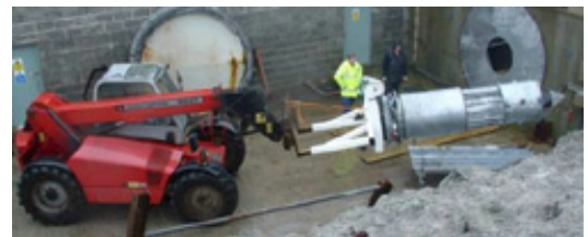
small turbine being installed on Limpet for testing.
