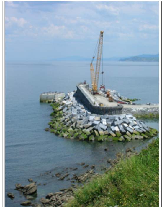
Construction site of the new breakwater in Mutriku’s harbour
